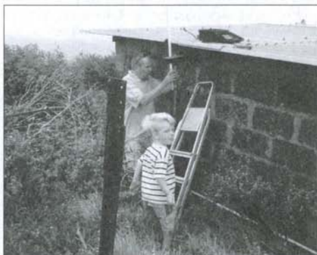
ZD8I Ian and his son Simon installing the new vertical for the ZD8VHF 6m beacon on April 23, 2006
